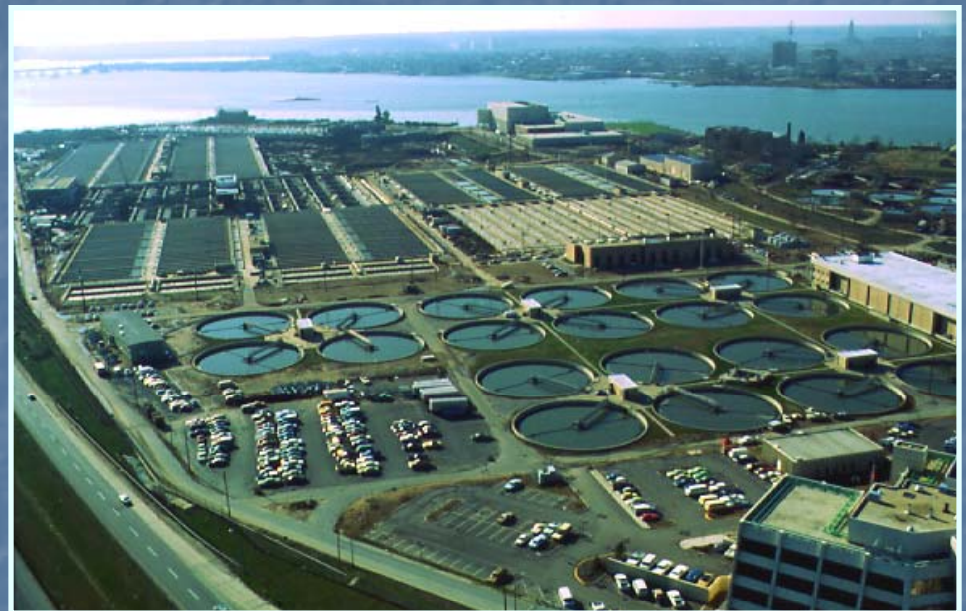
Blue Plains Advanced Wastewater Treatment Plant
